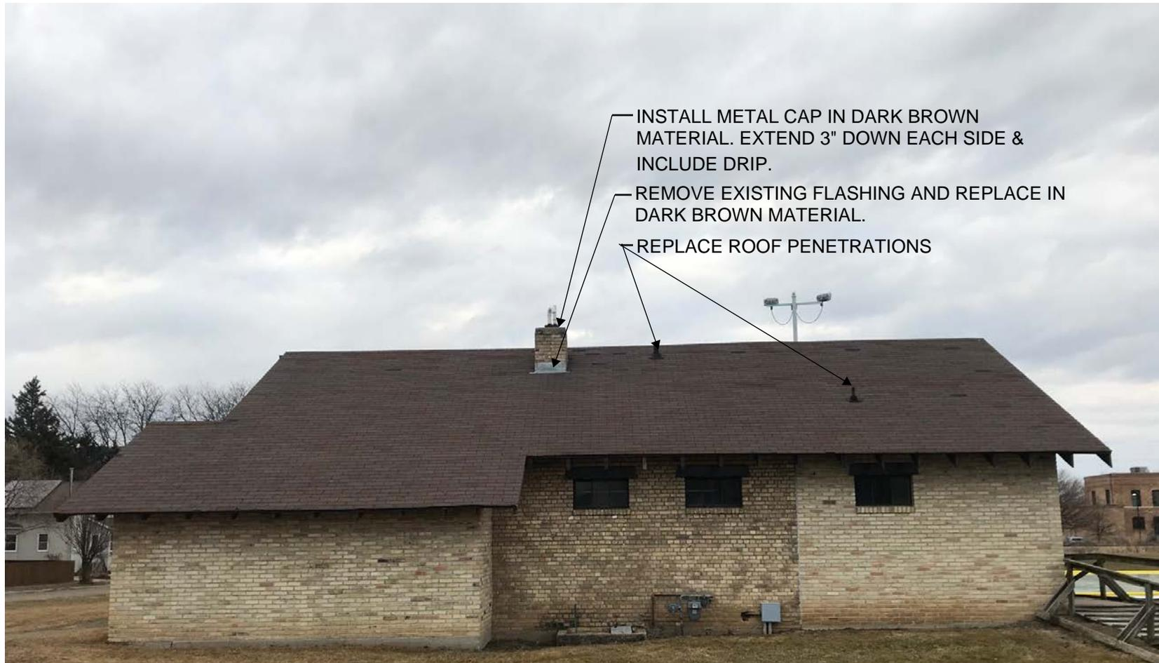
INSTALL METAL CAP IN DARK BROWN MATERIAL. EXTEND 3" DOWN EACH SIDE & INCLUDE DRIP.
